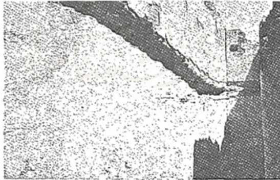
Pl. V. The holes where the bars of the wooden Coridor of the upper story of the entrance are still in situ.
